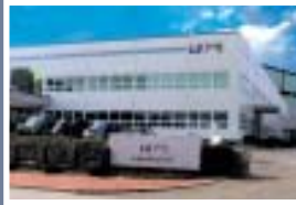
Dalian Plant (China)
